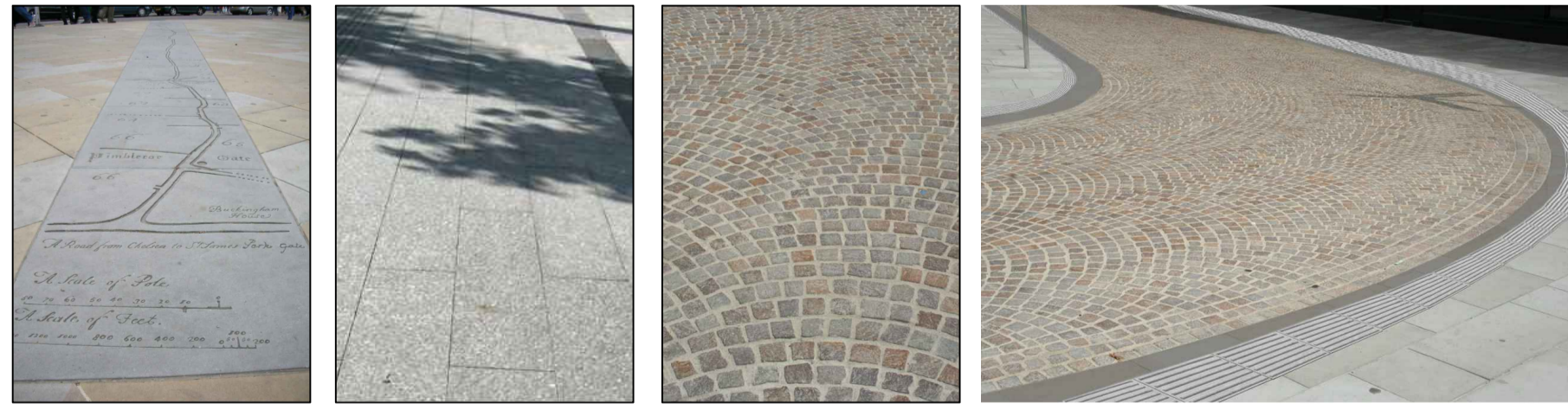
Example of Inlaid Artwork recessed within paving Example of Natural Stone paving to footpaths Example of Natural Stone Feature Paving Example of Natural Stone Paving to Restricted Access Road only, with flush stone kerbs and contrasting stone tactile paving
